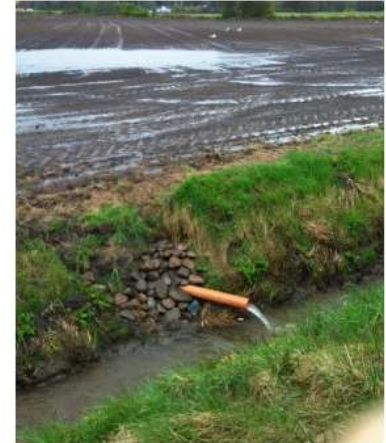
Figure 3. General sketch of agricultural drainage and an example of subsurface drainage entering a drainage ditch. Illustration: Johan Kling
